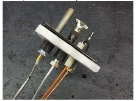
12. Lower the new pilot assembly into position with the Thermopile (the tall cylindrical component of the pilot assembly) toward the front of the Fireplace and the pilot hat jets directed toward the burner pan. Gently bend the lines back toward the back of the stove.
